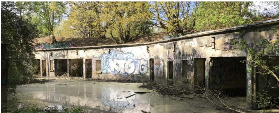
North Weald Redoubt Scheduled Monument
